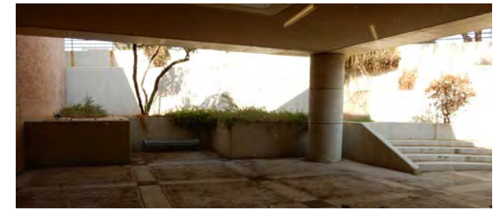
East sunken courtyard accessed from Library Children's Section
