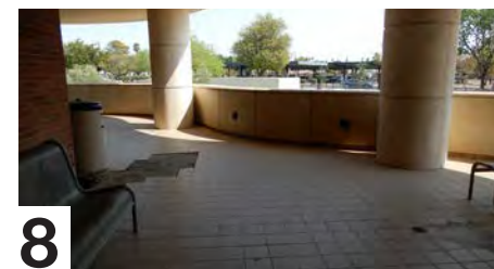
8 Staff balcony is underutilized
