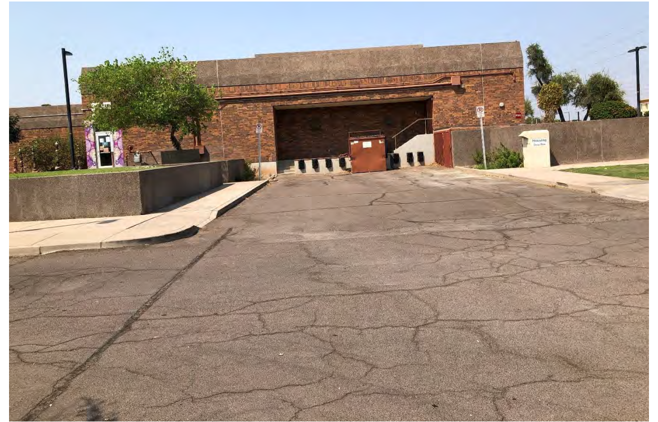
Photo 3 – South Elevation at Loading Dock
