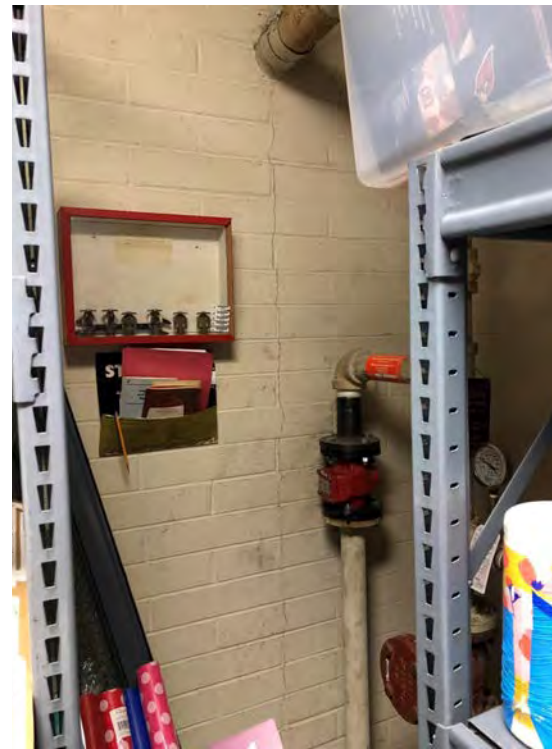
Interior Masonry Crack
