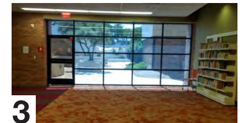
3 Natural light and emergency egress afforded by sunken courtyards
