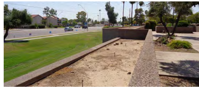
Planter walls along Rural Road east of the Edna Vihel Arts Center
