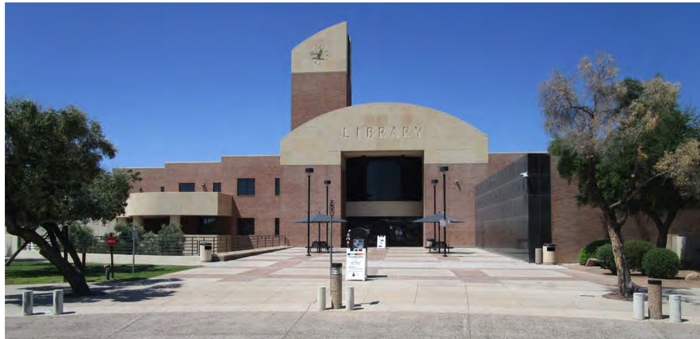
Main library entrance and drop-off area.
