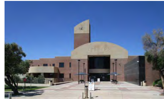
Tempe Public Library Front Entrance
