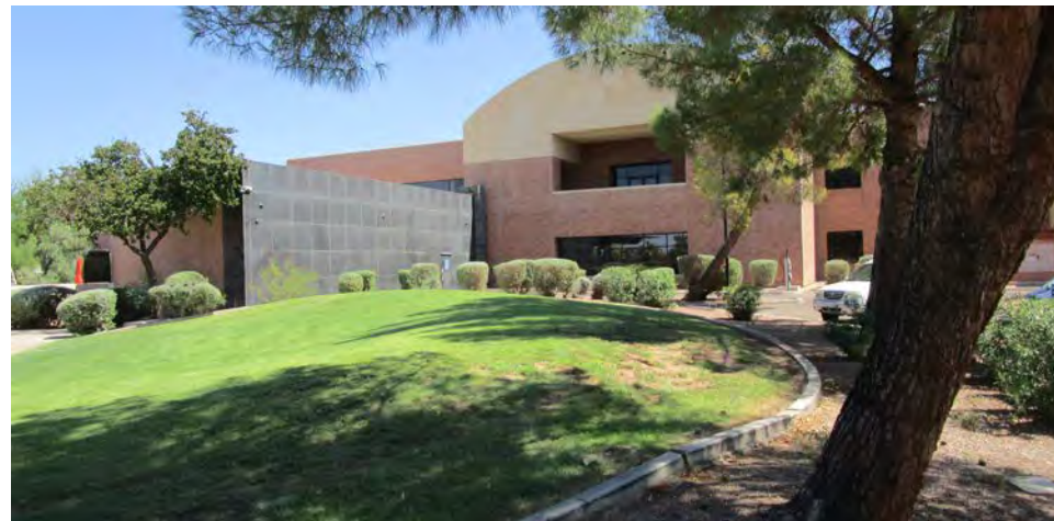
Library "Back of House" contributes to deactivation of north campus
