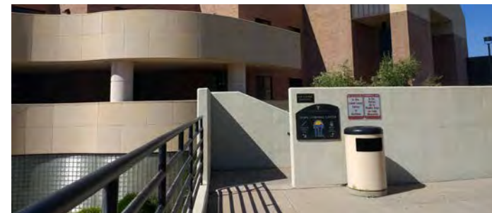
Unsecured exterior stairway leading to south sunken courtyard
